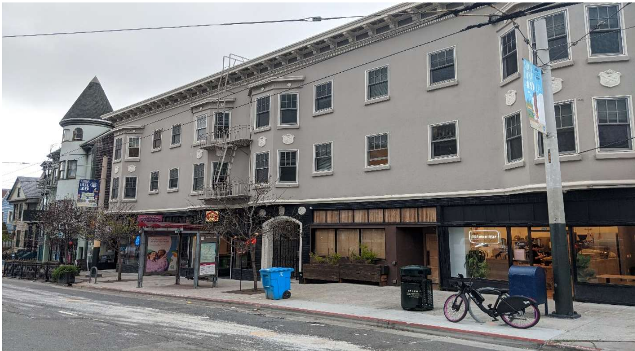
Figure 5. 'Shaken' Small Businesses at Divisadero Street and Haight Street. Prior to retrofitting, this building housed two smoke shops, a café, and three family-owned restaurants: a burger joint, a pizza-by-the slice counter, and a Korean sandwich shop. After retrofitting, only the pizza restaurant remains. An artisan coffee and tea café, 'Instagram-ready' bubble tea shop, sit-down sushi restaurant, and 'fusion' Indian wine bar now occupy the other spaces (Week, 2020).
