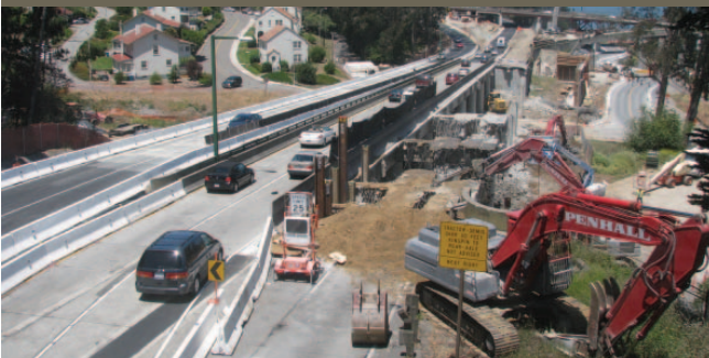
STAGE 3: Demolition of Old Bridge
